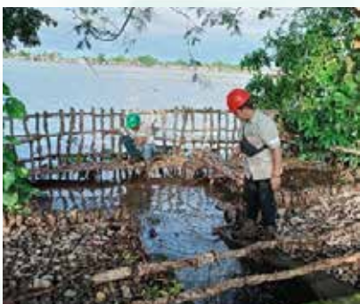
Pembuatan Siring Sungai Construction of River Siring (Gabions)
