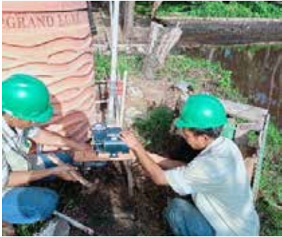
Perbaikan Mesin Pompa Air Water Pump Machine Repairs
