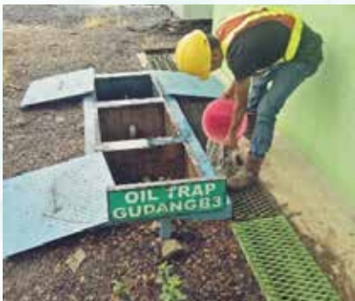
Perawatan Oil Trap Oil Trap Maintenance
