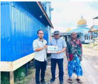
Pembangunan gudang di Masjid Ar Raudah, Desa Banua Anyar Construction of a Warehouse at Ar Raudah Mosque, Banua Anyar Village
