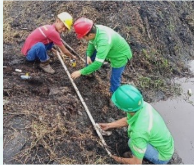
Perawatan Pipa Settling Pond Settling Pond Pipe Maintenance
