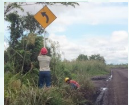
Pemasangan Rambu-Rambu Area Hauling Installation of Hauling Area Signs
