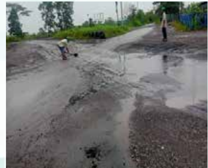
Perawatan Jalan Kampung Village Road Maintenance
