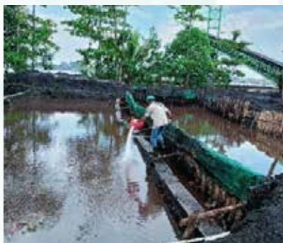
Pemberian PAC pada Settling Pond PAC Application in Settling Pond
