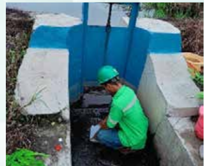
Perawatan Pintu Settling Pond Settling Pond Door Maintenance
